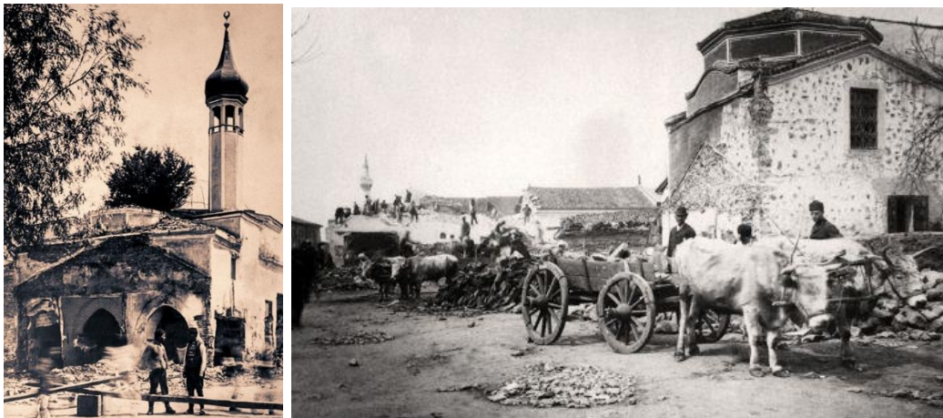
Figure 5 (left): The demolition of the Keremetian Mosque dated to the second half of the 19th century (Photo archive: NAIM-BAS)
