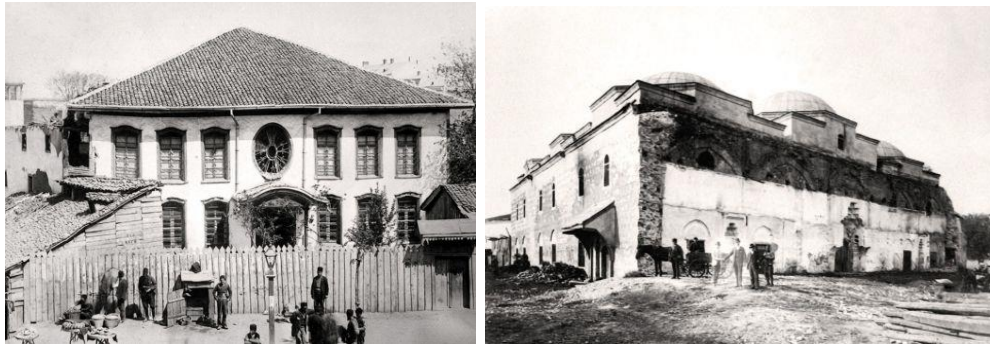
Figure 7 (left): The Nuri Pasha House, demolished after 1877-1878 (Photo archive: NAIM-BAS)
