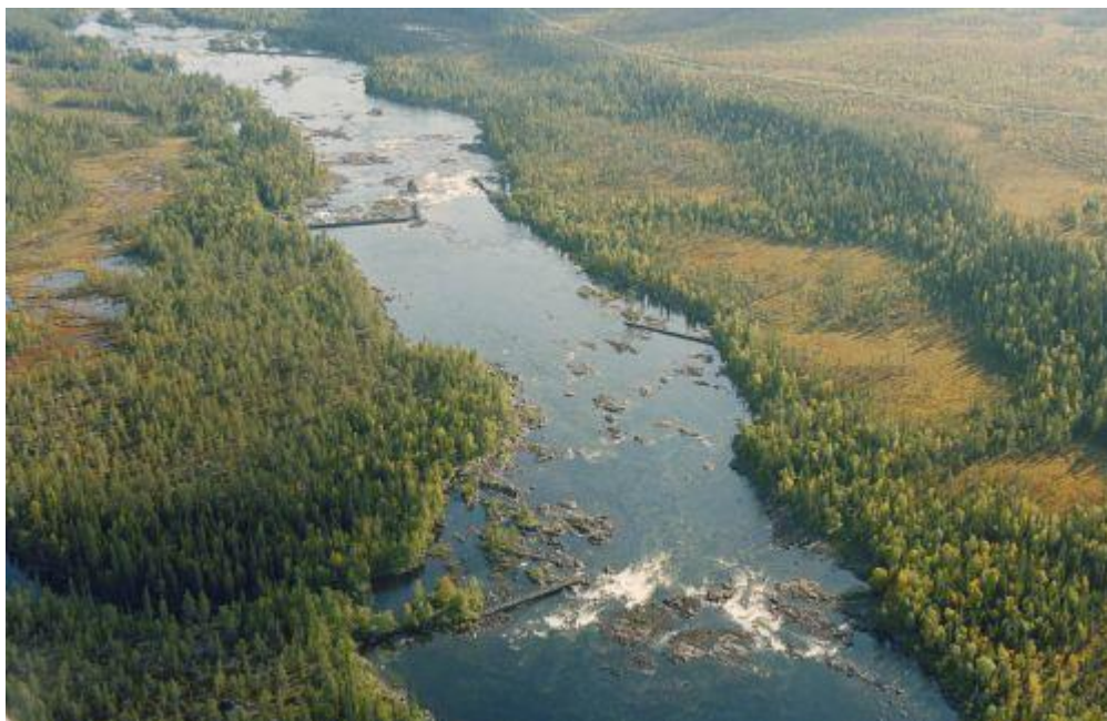
Figure 2: Constructions in Laisälven built for log driving. Photo: Jan Norrman (Creative Commons Attribution 4.0 International License)
