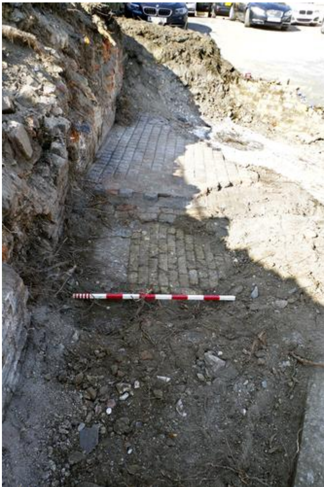
Figure 37: Yellow brick surface 1213, red brick wall 1210 and later textured concrete surface 1211. 1 x 1m scale. View from east
