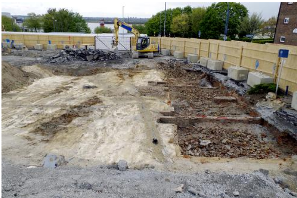
Figure 39: Cellars 1036=1112 and 1113-1117 fronting Queen Street. 1 x 1m scale, 2 x 2m scales. View from south
